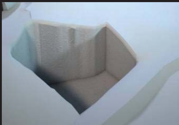
1 st step - Excavation
