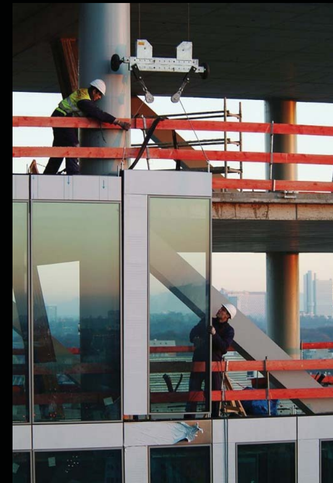
Fassade assembly using monorail system (example)
